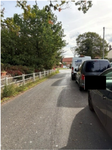
Picture of the Street looking towards war memorial showing railings protecting road from stream and the vehicles parked along it.
